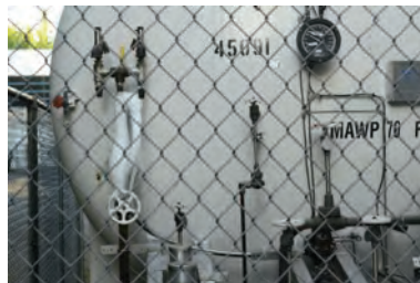
Difficult inspection sites
